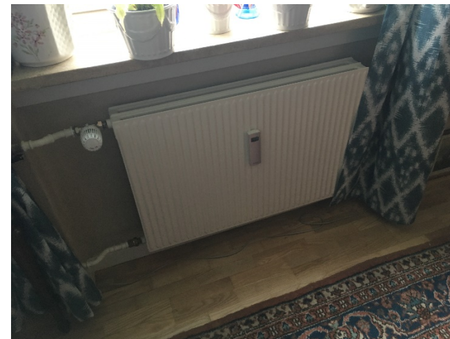
Radiator i stue
